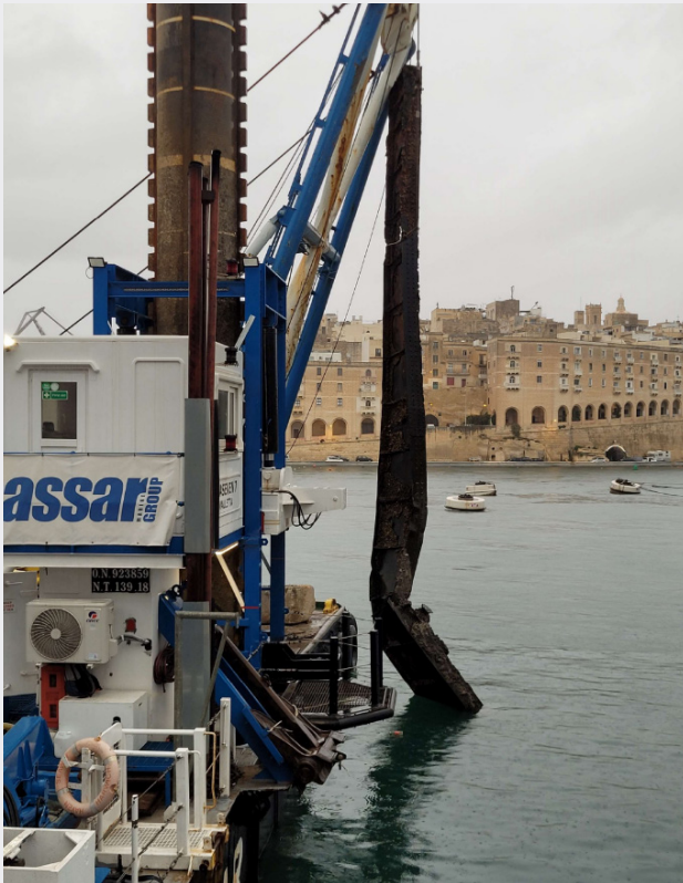
Crane lifting a metal structure during works at Fort St Angelo.
