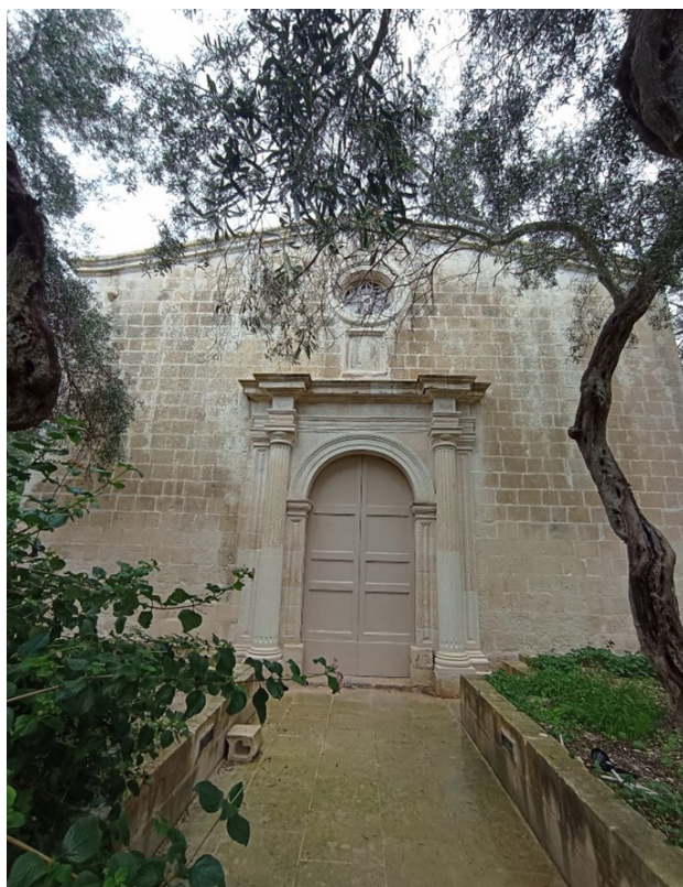
Façade of the Old Parish Church Tas-Salvatur, Lija.
