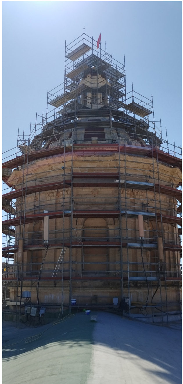
Dome of St Paul's Basilica under restoration.
