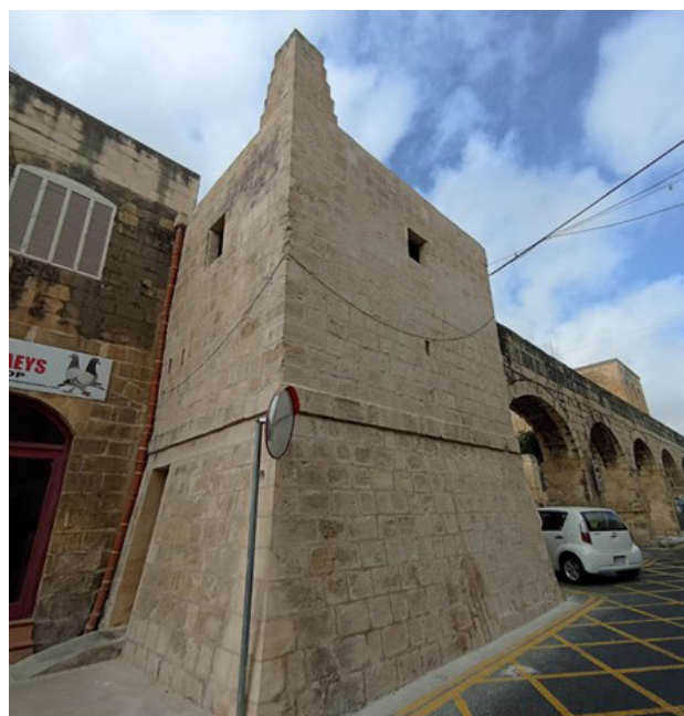
Wignacourt Aqueduct Water Tower after restoration.
