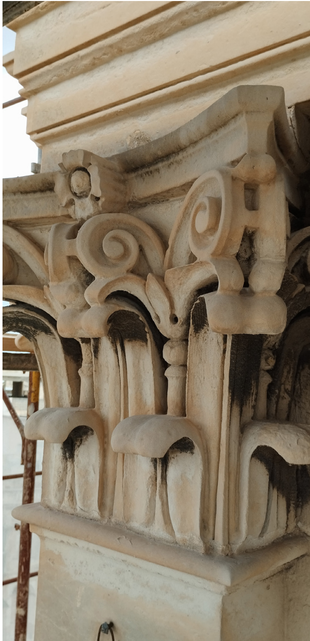
Detail of restored pilaster, Holy Trinity Church, Marsa.
