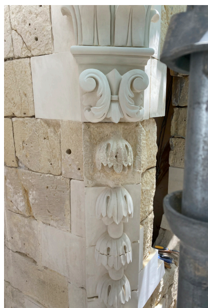
Detail of restoration works showing recovery of lost decoration on St Paul Niche.
