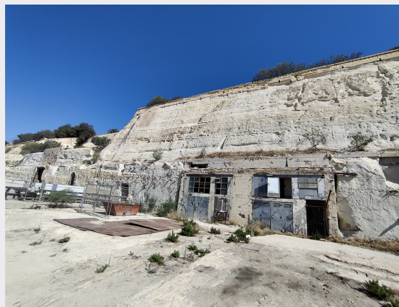
Marsa rock-cut powerstation.
