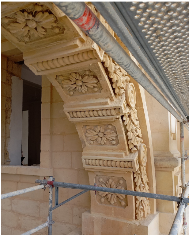
Newly cleaned decorative element on the main façade.
