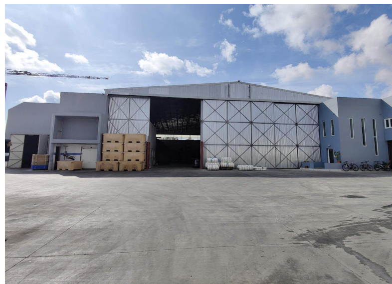
Seaplane Hangar, Marsaxlokk.
