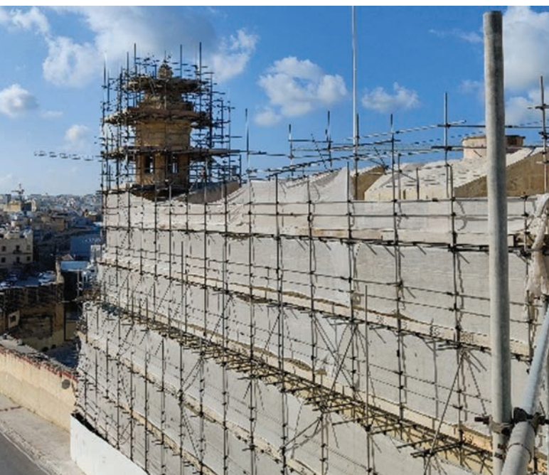
Senglea Land Front – Restoration works during 2020/2021.
