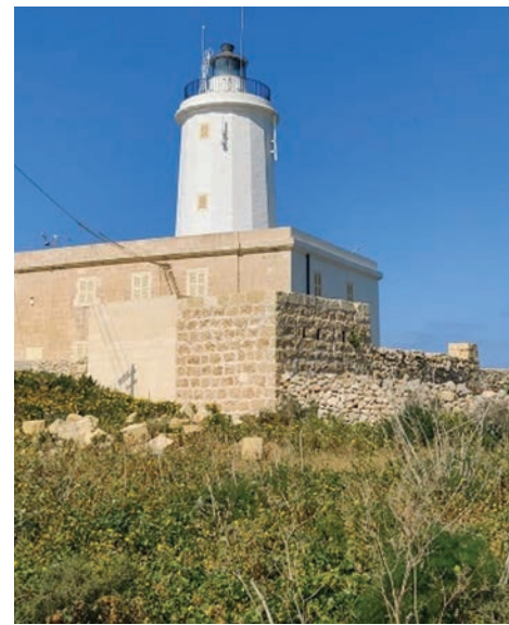
Ta' Ġordan Lighthouse - restored facades.
