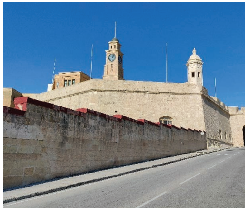
Senglea Land Front – Completed restoration works.
