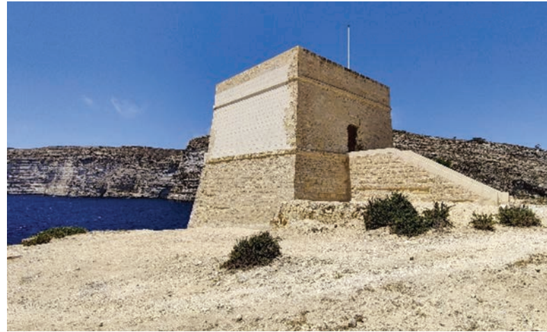
Munxar Tower – External restoration works.
