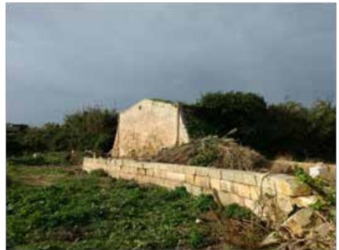
View of the back façade (south-east) of the Chapel of San Mikiel is-Sanċir
