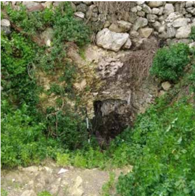
Entrance to the underground complex-external Image: Superintendence of Cultural Heritage
