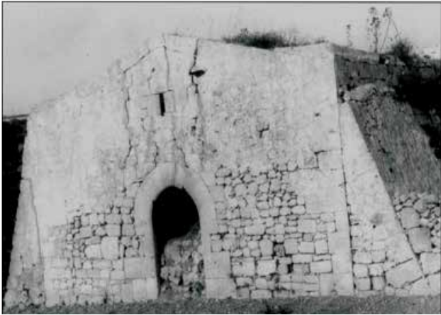
View of the front façade of the Chapel of San Mikiel is-Sanċir in c. 1968 before restoration works carried out in the 1970s. Note the buttresses aimed at providing support to the structure. The buttresses are eighteenth century additions.
