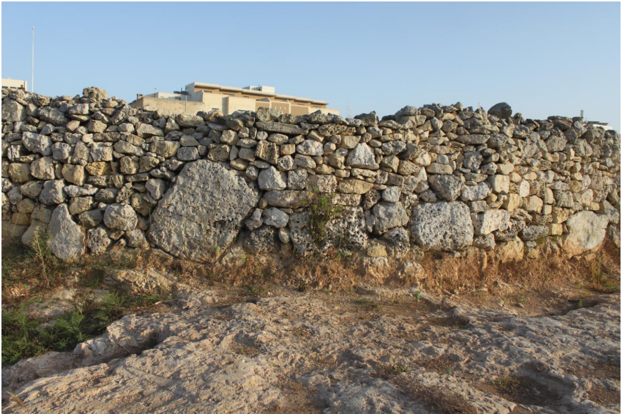
Plate 8 – Large ashlar blocks within various stretches of the rubble walls
